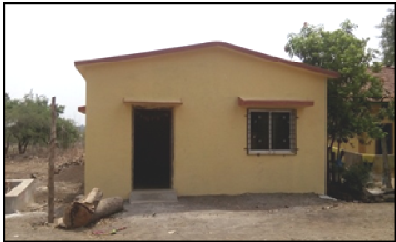
New Anganwadi building at Savroli.
