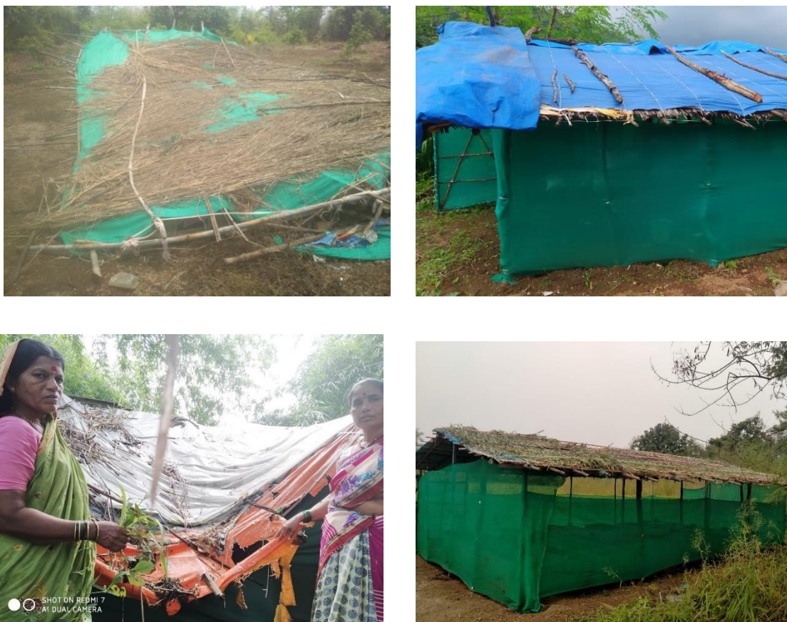
Figure 38 (L to R) Ambarpada and Kalgaon Before and After Shed Rebuilding
