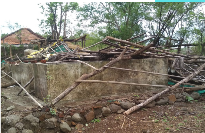
Khoste VC shed
