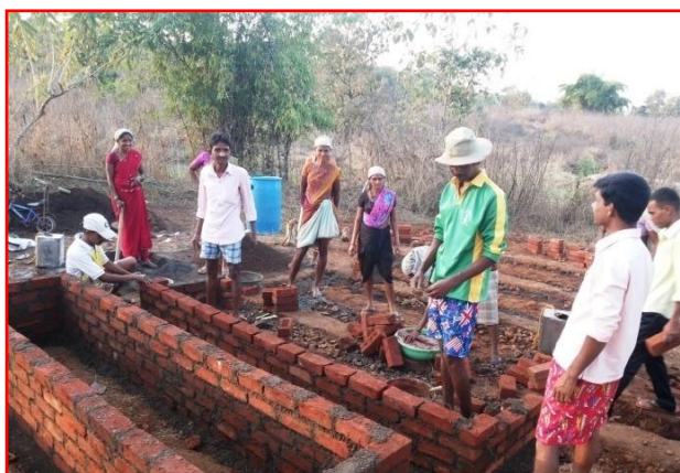
Construction of pits in progress at Ambivali (left)
